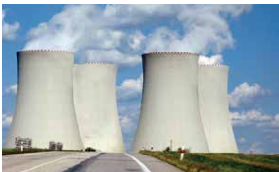
Power plant flue gas desulfurization and denitration
