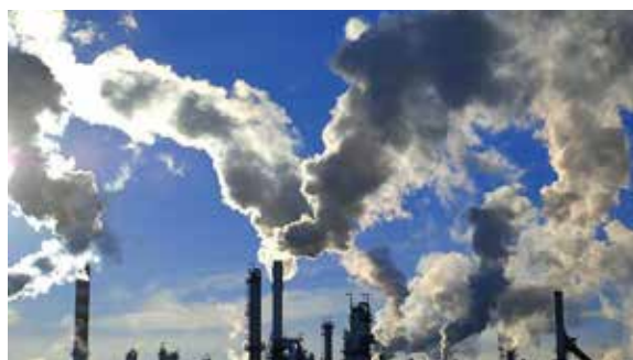
Cement plant flue gas desulfurization and denitration
